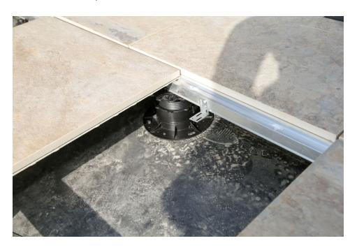
**Step 11:** For non-perimeter rows, use and Mbrico T-Track so tiles can be received on both sides of the track. This provides automatic spacing and captures the tiles.
