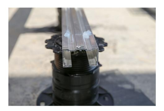
**Step 12:** When installing, check that the laid slabs are level using the slope adjustable feet. Supplied shims can be used if additional slope correction is needed. Set laser and tripod on top of tile to insure level installation.
