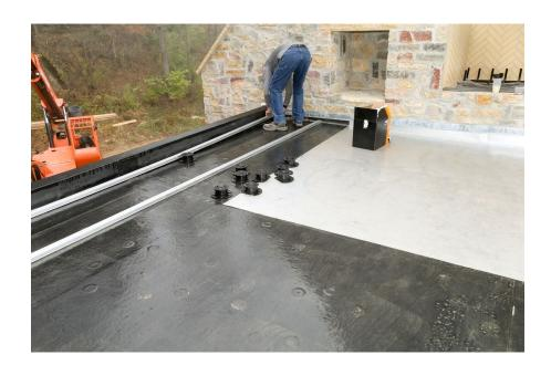
**Step 5:** Using your provided surface plans, begin placing pedestals spaced accordingly to load requirements. (See image below).
