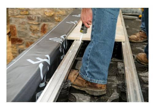
**Step 8:** Tiles are to be adhered to perimeter track and overlap to compensate for distance between wall and pedestal. Leave at least 1/8" gap between tile and structure.
