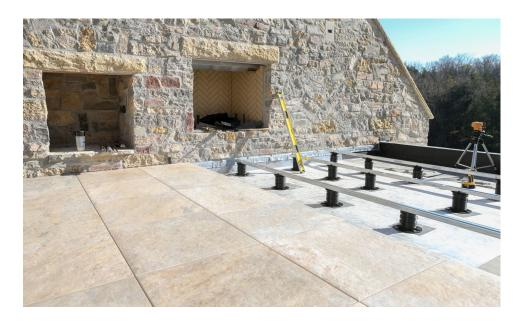
**Step 17:** When opposite perimeter is reached and final row is to be installed, tiles can be cut to size to meet dimension requirements. Tiles can be cut using a conventional wet tile saw with a diamond blade.
