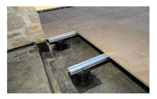
**Step 18:** Use Mbrico perimeter flat track to finish final row against structure. A 1/8" gap should be left between Mbrico surface edge and any structure or wall to allow for proper drainage. See step 7.
