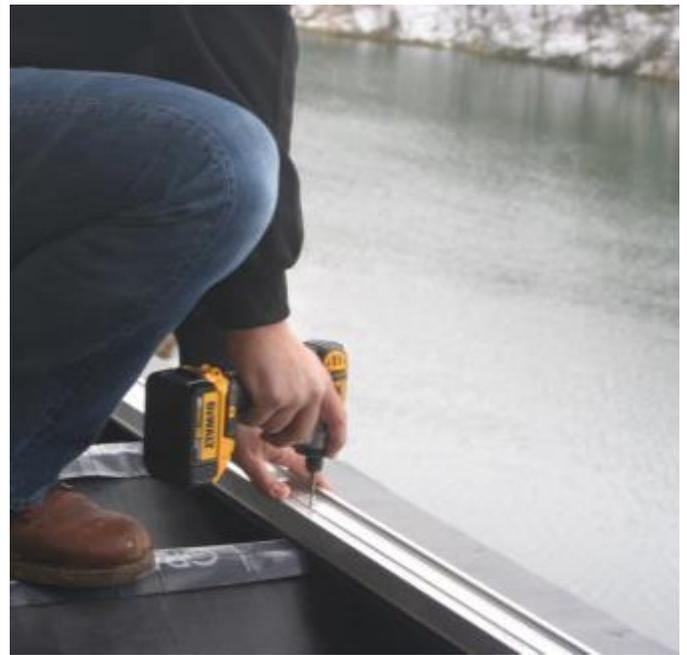
**Step 6:** Using a single tile as a spacer, place the tile groove over the male spline on your starting track. Place several tiles along the length of your track piece, these will serve as a guide for your next 2-sided track.
