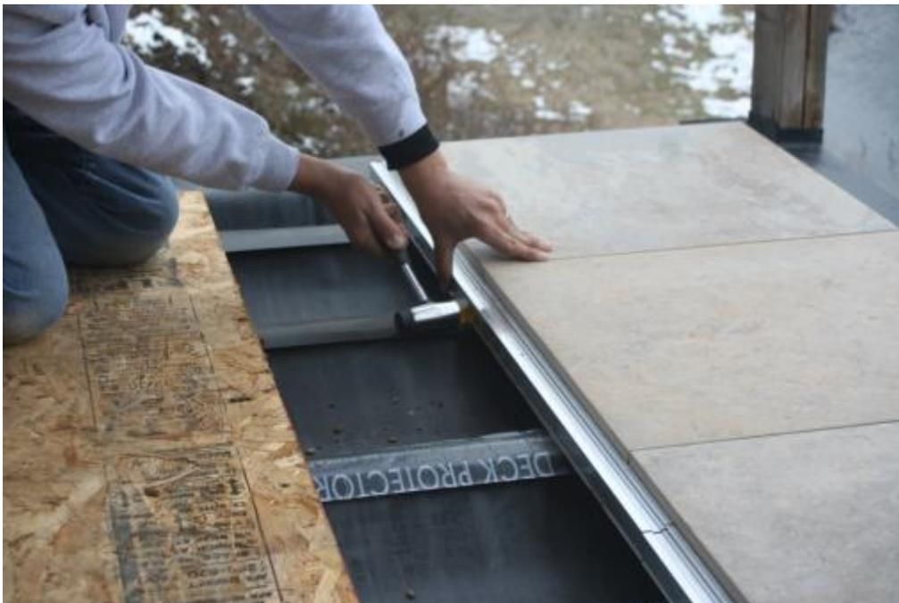
**Step 9:** Repeat steps 1-8 until last row then using a single sided track at edge slide final row of tiles in from end.
