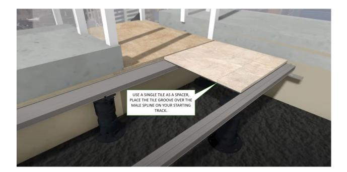
9. Continue to place tiles on the track. Create a snug fit between the groove on the tile and the spline on your first starting track.
