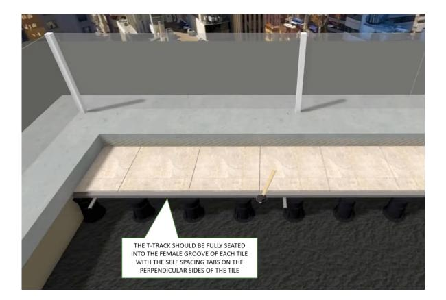
11. Check to make sure all tracks are fully seated into both grooved tile edges and that all tile gaps appear even and square. It is now time to attach the remaining end of the cross brace channel which is still exposed.
