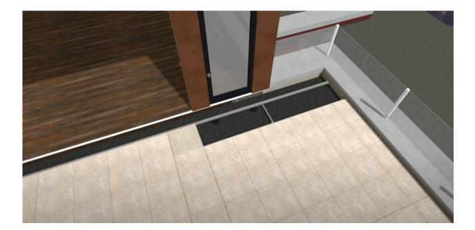
14. On your final row, cut tile to size if needed and regroove any edges that will engage with track (see separate instructions for cutting and regrooving). Small spaces can be left between tiles temporarily so that final cross brace connectors can be attached. Once cross brace connection are attach tiles can be tapped into final snug fit using a rubber mallet.
