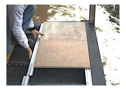
**Step 7:** Lift the tile sliding the next track into place sideways. Align your pre-drilled holes to your deck joist. Install 1 screw at each joist securely but not over tightened.
