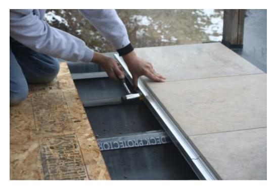
**<u>Step 9</u>**: Repeat steps 1-8 until last row then using a single sided track at edge slide final row of tiles in from end.
