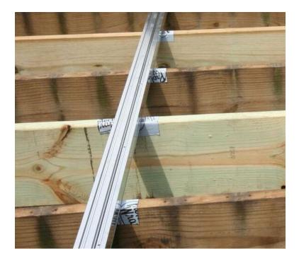
**Step 5:** Place a single sided rail per your layout at your designated starting edge. Once you have positioned the track piece, pre-drill a hole using a 3/16" drill bit at all points where the rail will intersect the deck joists. Secure track to joist using stainless screws provided. Snug securely, do not over tighten causing track to warp. Make sure the track stays square to your deck.
