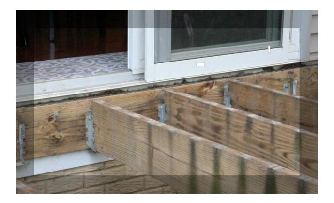
**Step 2:** Make sure the deck frame is square and relatively level. Any individual joists or framing surfaces that are crowned upward need to be planed down to level of the entire deck framing height.
