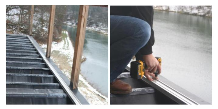
**Step 6:** Using a single tile as a spacer, place the tile groove over the male spline on your starting track. Place several tiles along the length of your track piece, these will serve as a guide for your next 2-sided track.
