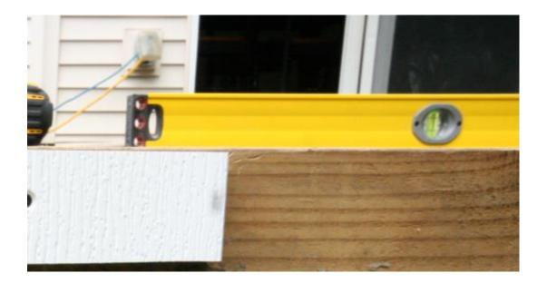
**Step 4:** After the deck framing is leveled, place the protective tape provided with your order, at all points where the aluminum track will contact your deck joists. Make sure the adhesive side of the tape is evenly and securely applied with no wrinkles against the joist.
