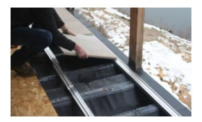
**Step 8:** Move any of your spacer tiles as necessary to place screws. Install all tiles in that row before starting on next. A rubber mallet may be used for sliding the track into the machined groove in the tile. Always check for square and parallel to structure and finish row.
